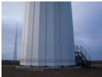
[Siemens' Bolted Steel Shell Turbine Tower](#)
