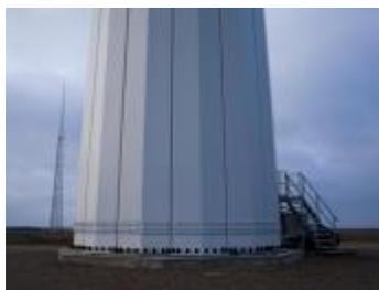
[Siemens' Bolted Steel Shell Turbine Tower](#)
